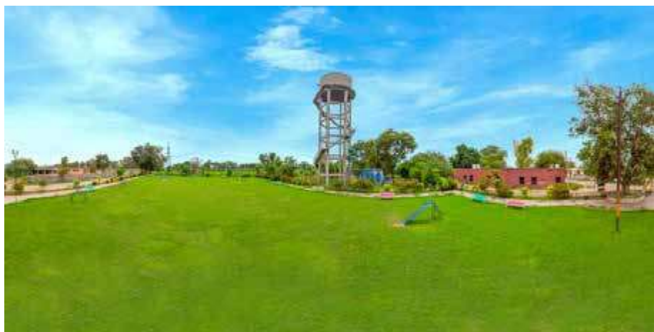
One among the 1700 community water purification units deployed in India using AMRIT technology.
